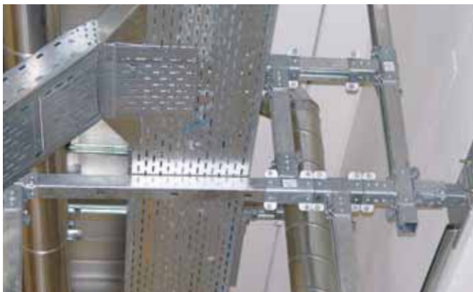
Typical application of the HALFEN System: Anchor and framing channels with POWERCLICK and framing fittings
