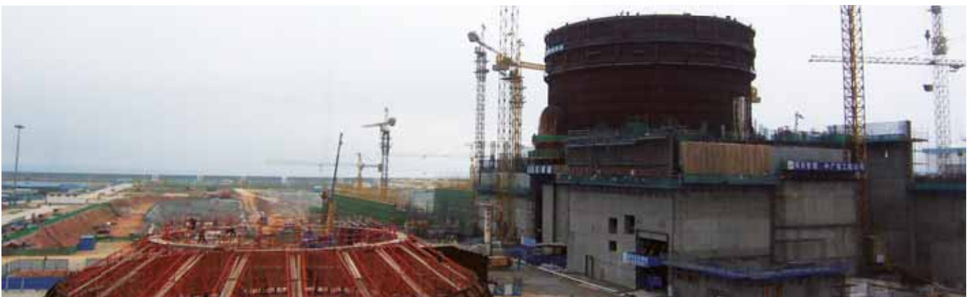
Nuclear power plant under construction
