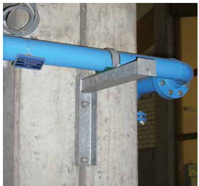
Cantilever fixed to vertical serrated channel for pipe support
