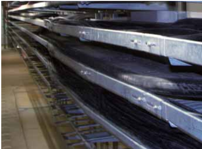
Stacked cable trays fixed to vertical serrated channels
