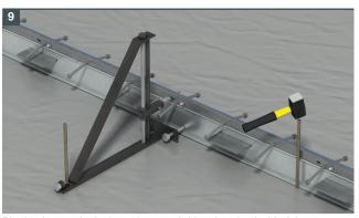
Pin the ArmourJacks into place and drive the pins behind the ArmourJoint in between the jacks.
