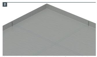
Measure the distances to the walls and edges. Set up the string line following the joint location.
