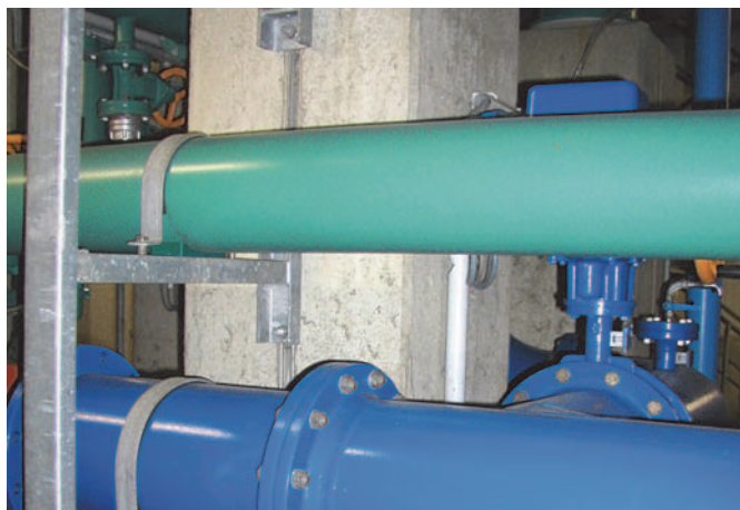
Pipe supports on vertical HZA Channels
