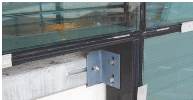
Fixings for curtain wall façades
