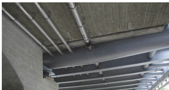
Fixings for drainage systems
