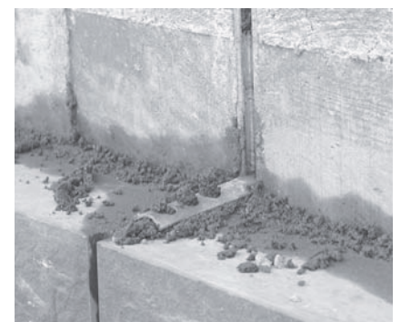
ML/BL Masonry connection
