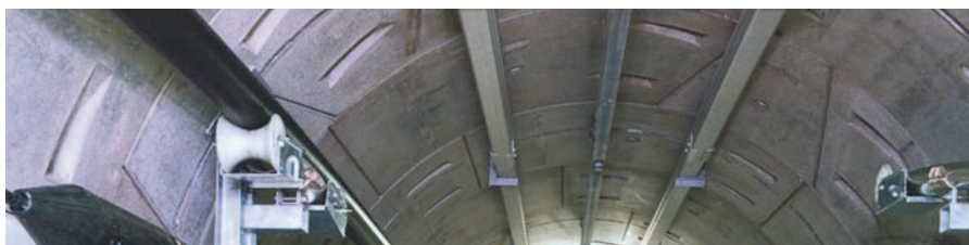
Curved HALFEN Cast-in channels in tunnel segments
