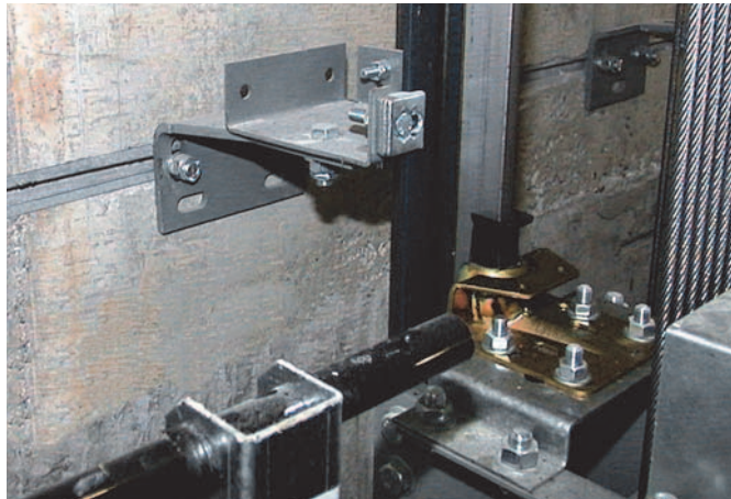
Fixing for guide-rails
