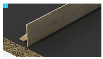
Flick a chalk line along the form board at the centre of the slab thickness.
