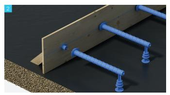
Nail the face fixing caps onto the form board using nails. Insert sleeves onto the fixing caps prior to pouring the concrete. To make the job easier the sleeves can be installed after the reinforcement has been laid and chaired. The face fixing caps can also be screwed to steel formwork using self-drilling screws.
