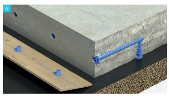
When concrete has hardened, the form board can be stripped to expose the open end of the sleeves.
