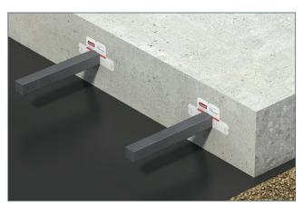
**Step 5**Firmly place the square dowel into the insertion hole in the flange dowel box by punching through the sticker as shown above.
