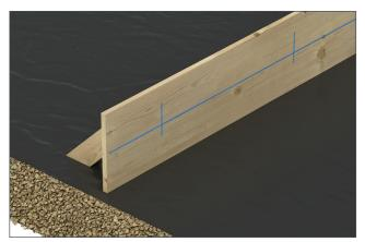
**Step 1**Mark centre line of the Connolly Flange Dowel Box and dowel spacing on the formwork. Flange Dowel Box is normally installed at the mid-height of the slab.
