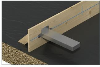
**Step 2**Place the Connolly Flange Dowel Box at the marked location by using the V-Notches at the top and both sides to ensure correct placement.
