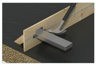
**Step 3**Nail the Connolly Flange Dowel Box to the formwork using three nails.
