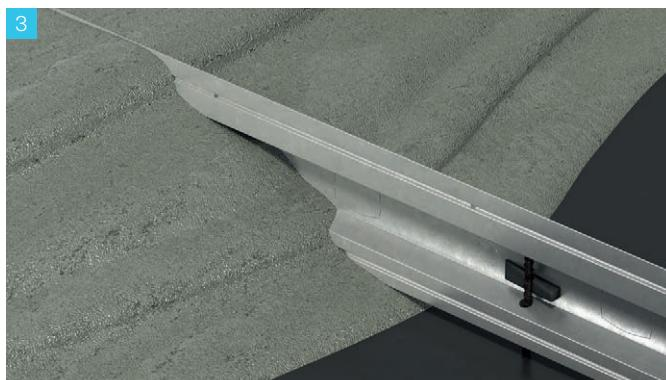
Place the reinforcement and pour the concrete over the key joint. Finish concrete surface to the top of the joint (**not above it**). Always pour concrete evenly to both sides of the joint and ensure concrete is compacted into the keyways.
