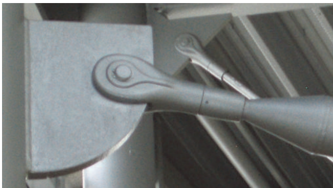
Compression system connected to a welded plate
