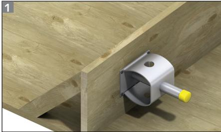
1 Nail the sleeve component to the formwork ensuring that the sleeve is correctly orientated for the direction of the load. Check that the minimum spacing and edge distances are not exceeded. The label prevents debris from entering into the sleeve aperture and should not be removed at this stage.
