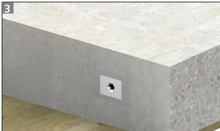
3 When the concrete has achieved sufficient strength, strike the shuttering. Peel off or puncture the label to reveal the hole for the dowel. Where HSD-V or HSD-ULTRA-V are being used, the label should only be punctured enough to allow the dowel into the cylindrical sleeve.
