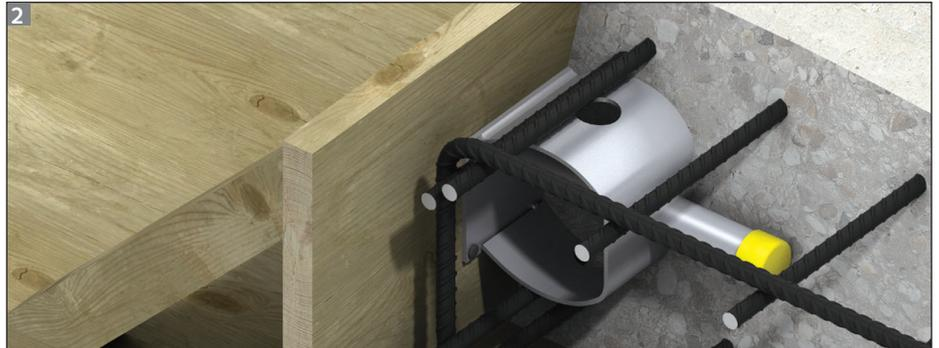
2 Fix the local reinforcement in position around the sleeve component together with any other reinforcement that is required, ensuring that the correct cover to the reinforcement is maintained. Pour the concrete to complete the installation of the sleeve component.
