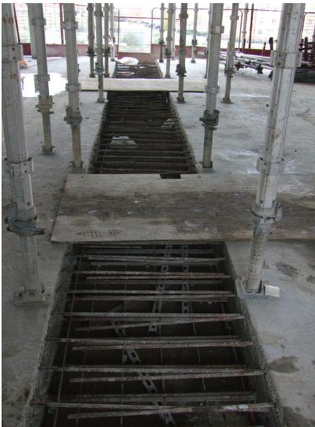
Pour Strips restrict site access, cause a trip hazard and delay progress on site
