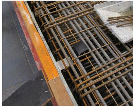
Reinforcement around HSD-LD-S 20 Sleeves
