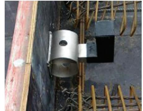
HSD-LD-S 30 Sleeve nailed to formwork
