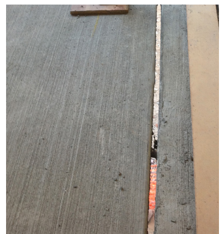
Finished slab using the Halfen HSD-LD
