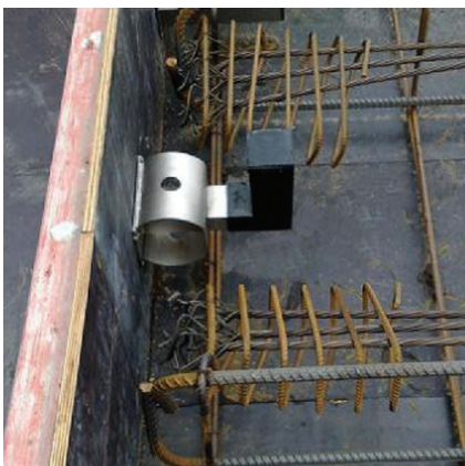
HSD-LD 30 Sleeve nailed to formwork
