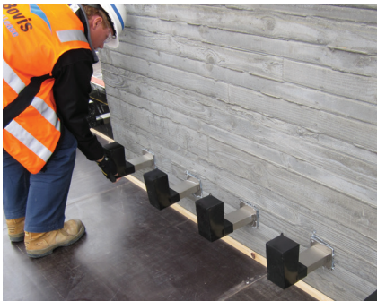
Sleeve pushed over dowel component at core wall
