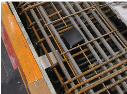
Reinforcement being located around HSD-LD 20 Sleeves
