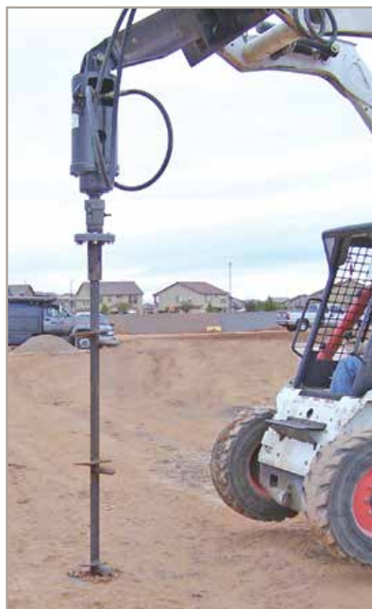
Typical MB Brace Badger Installation
