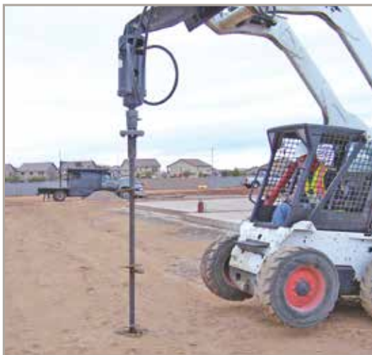
Typical MB Brace Badger Installation
