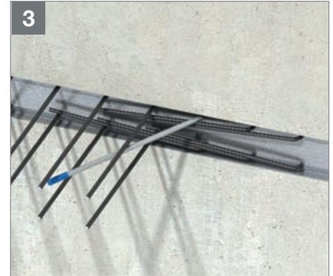
Attach the Keyway Box by nailing through the casing to the formwork or securely tie the projecting reinforcing bars to existing reinforcement. The Box should be firmly secured and tight against the formwork to avoid displacement during concrete placement.
