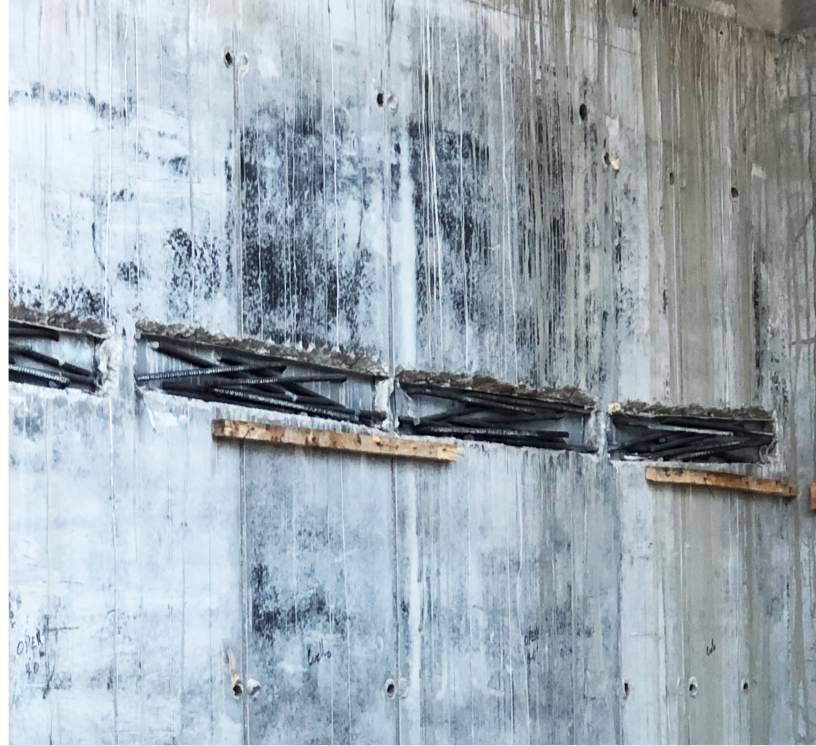
Left: MB Keyway Splice Box units are tied to the rebar prior to casting. Right: The KSB lid has been removed to reveal continuous reinforcing bars that will be bent outward and tied into the floor slab.
