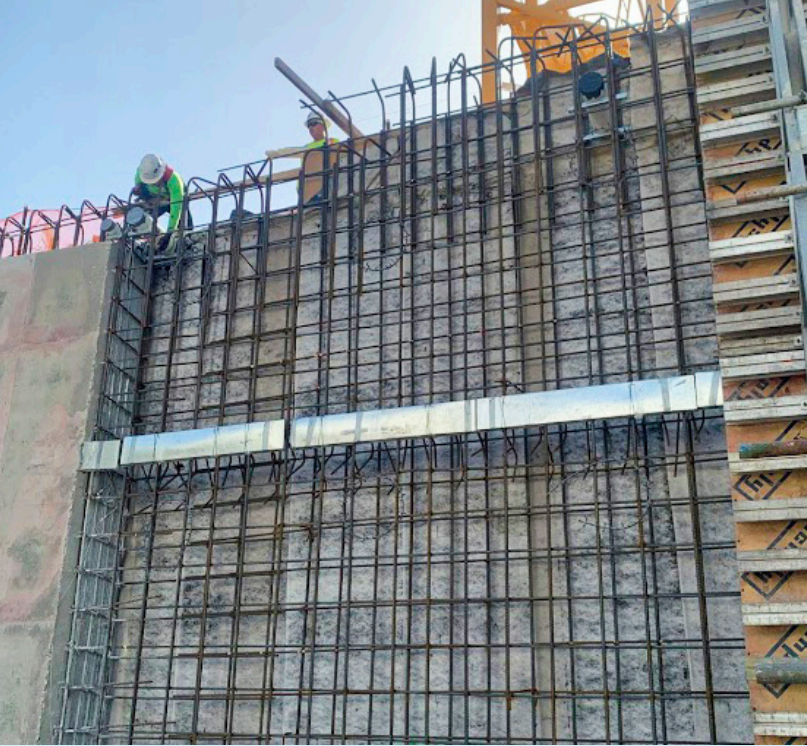
Left: MB Keyway Splice Box units are tied to the rebar prior to casting. Right: The KSB lid has been removed to reveal continuous reinforcing bars that will be bent outward and tied into the floor slab.
