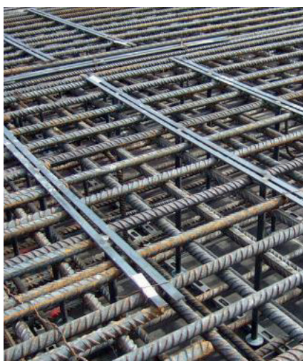
King's Dock Mill construction site in Liverpool, featuring the installation of the Ancon Shearfix punching shear reinforcement.
