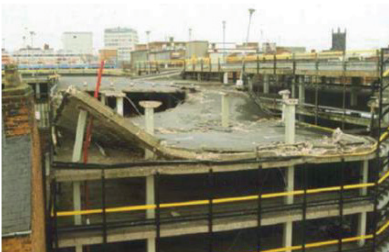
J.G.M. Wood, Pipers Row Car Park, Wolverhampton: Quantitative Study of the Causes of the Partial Collapse, SS&D Contract Report to HSE (1997)
