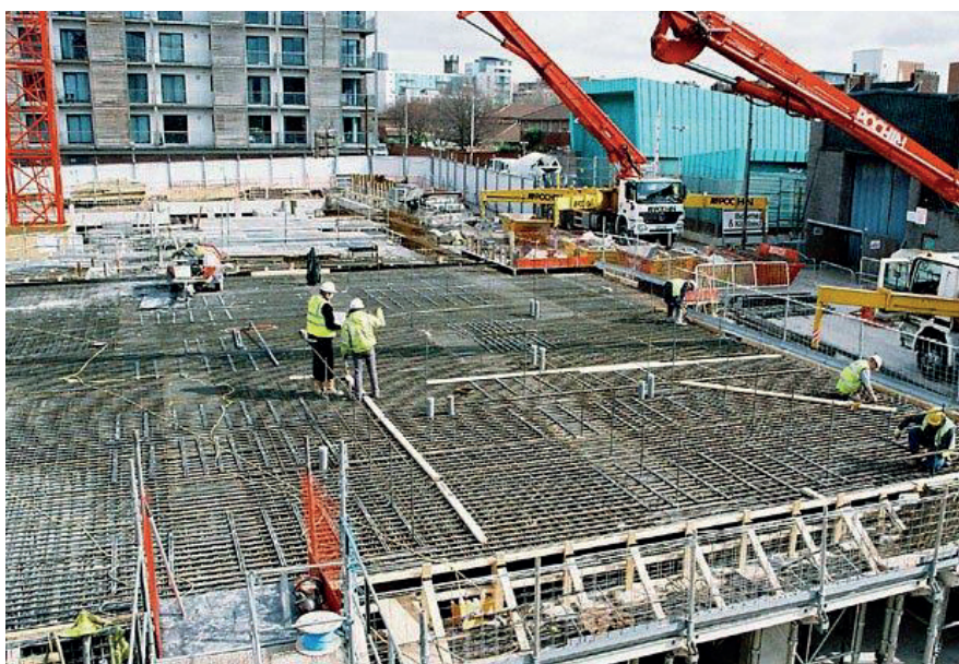
King's Dock Mill construction site in Liverpool, featuring the installation of the Ancon Shearfix punching shear reinforcement.
