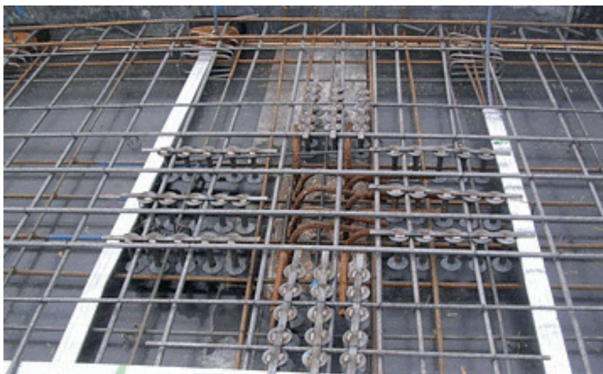
An Ancon Shearfix Punching Reinforcement system has been installed in a $1.5 billion waterfront development at Newport Quays, Port Adelaide.
