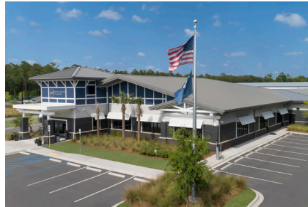
Berkeley Electric Cooperative Johns Island, South Carolina
