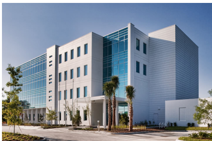
Toho Water Authority Kissimmee, Florida
