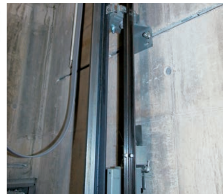
Elevator Guide Rail Connected using Cast-in Channels
