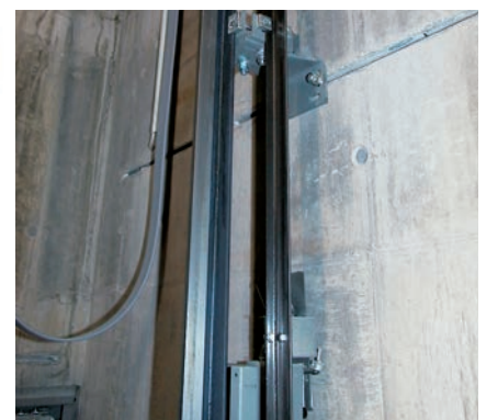
Elevator Guide Rail Connected By Anchor Channel
