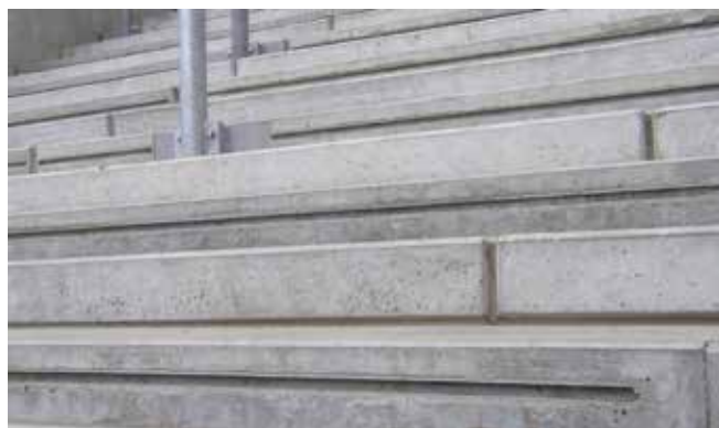
Bevestiging balustrade, statribune Rheinenergiestadion/Keulen
