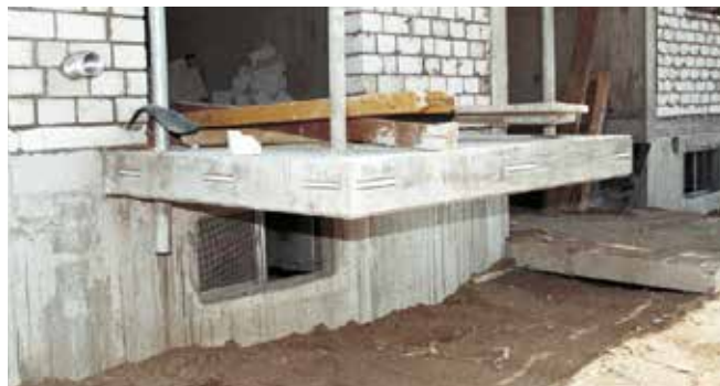
Ingestorte HGB rail, woningbouw
